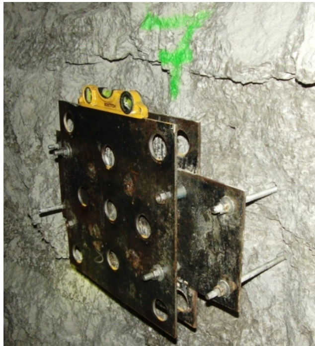
Figure 3.10. Mounted Drilling Template
